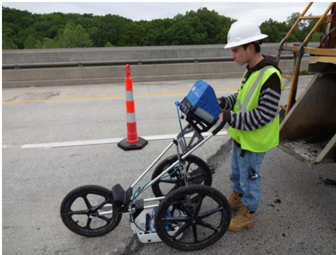
Figure 1. Ground Penetrating Radar Unit Scanning Bridge Deck
