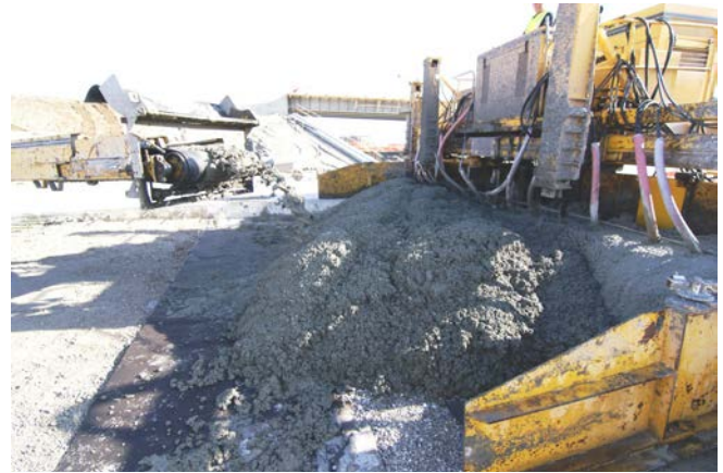
Figure 2. Casting pavement sections with RCA-made concrete
